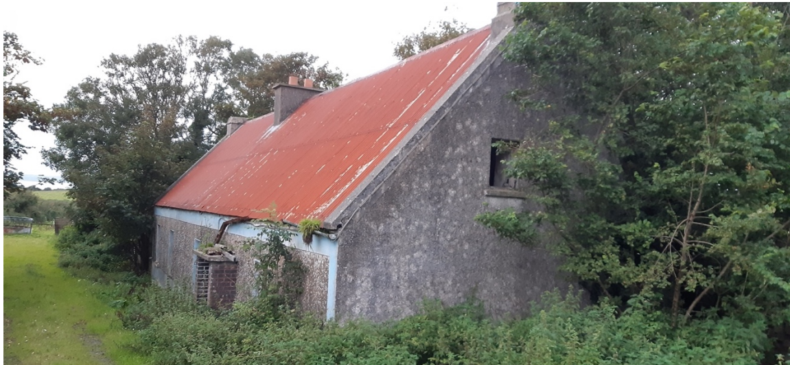
Photograph 37. (Location A, Building 2) with corrugated iron roof.
